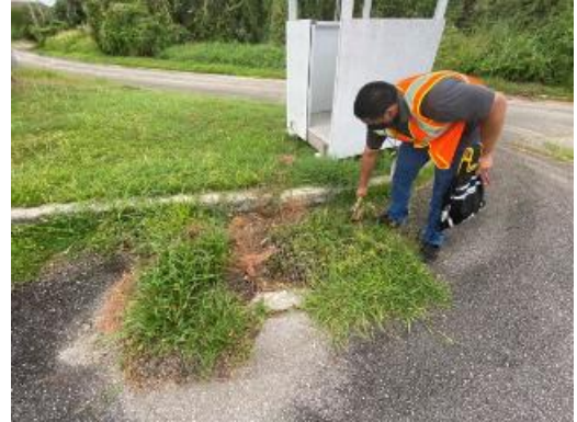
Figure 16 - Storm drain clogged with vegetation and debris at Inarajan ES
