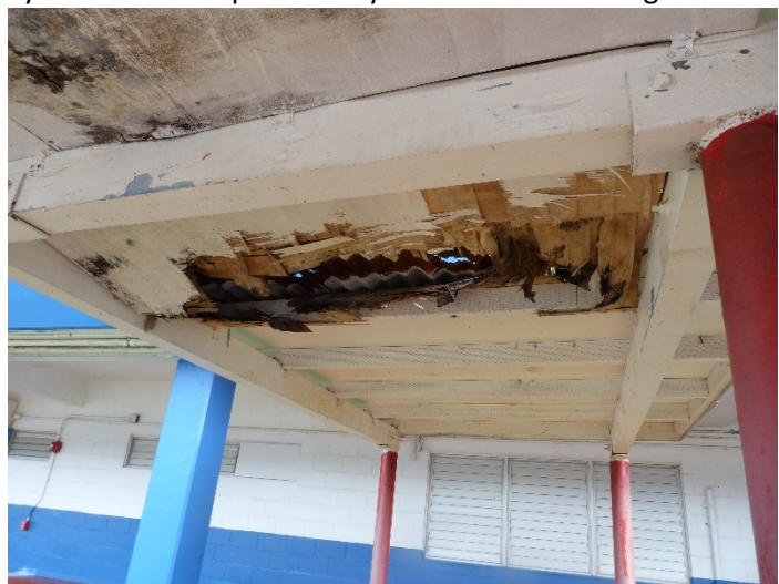
Figure 7 - Oceanview MS Walkway (23) wood roof damage.
