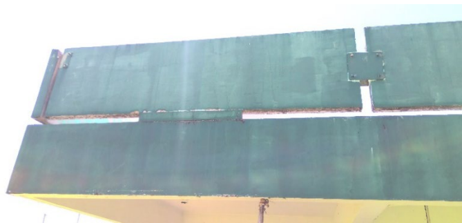
Figure 5 - P.C. Lujan ES Building 9 roof parapet - potential imminent collapse hazard
