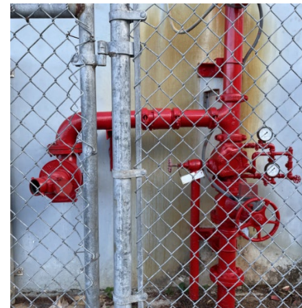
Figure 12 - Jose Rios MS sprinkler pipe leaks; system is shut down.
