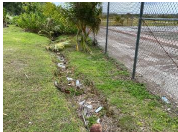
Figure 20 - Debris-filled drainage swale at Simon Sanchez HS
