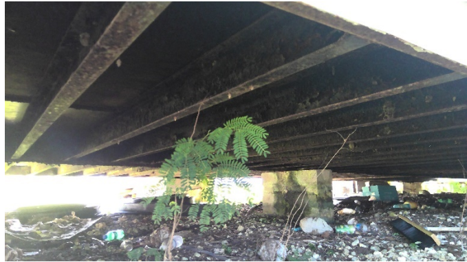
Figure 6 - Jose Rios MS B1 corroded steel floor joists and exterior beams
