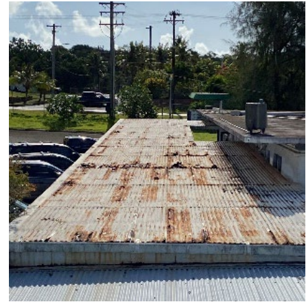
Figure 9 - Corrugated steel roofing rusting
