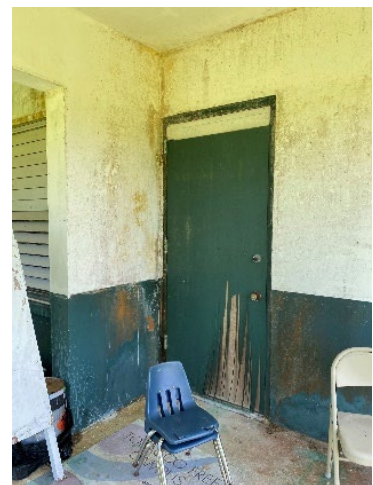
Figure 10 - Delaminating wood door
