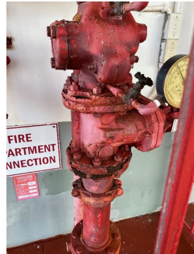
Figure 13 - Astumbo ES corroded fire protection infrastructure
