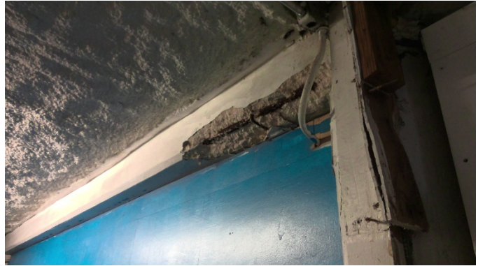
Figure 4 - Agana Heights ES Buildings 1 and 3 beam spall
